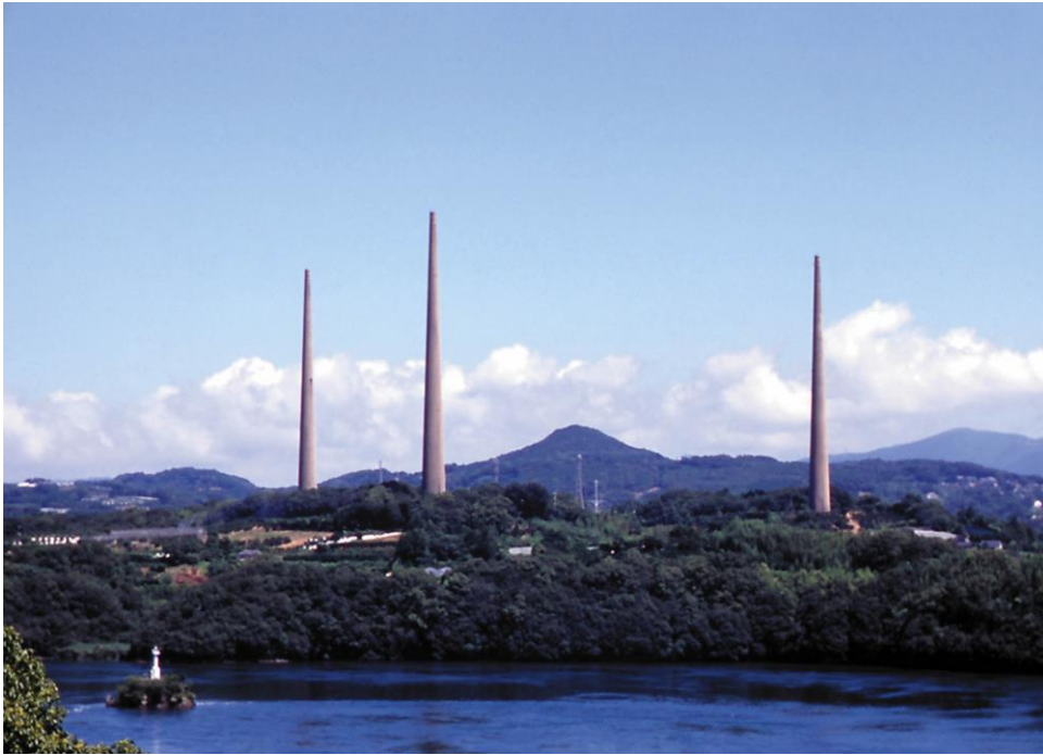
Fig.1 Old Sasebo Wireless Transmission Facility
